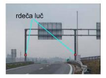
Figure 5: Warning signalization on exit ramp (left for correct-, right for wrong-way driving motorists)
