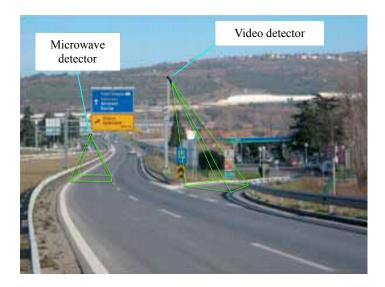
Figure 3: Microwave and video detection monitoring zones at H5 exit ramp to Trieste
